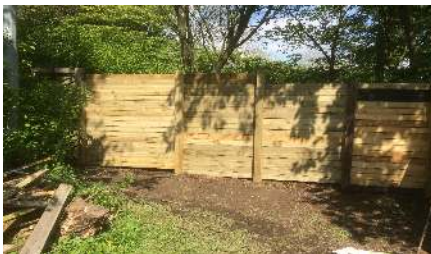
The newly refurbished fence in the Community Garden
